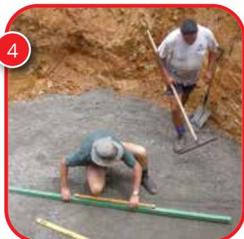
**4** Add 7mm Granular Fines as bedding material - this should be 75mm thick and be levelled in all directions with a straight edge and level.
