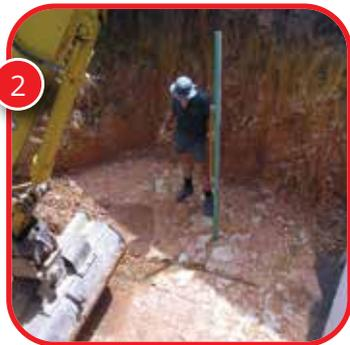
**2** The excavated hole should be square. The final hole size should be 4m x 4m x 1.2m depth
