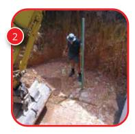
The excavated hole should be square. The final hole size should be 4m x 4m x 1.2m depth
