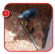
Level the ground which will form the base for your tank.
