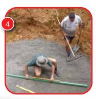
Add 7mm Granular Fines as bedding material - this should be 75mm thick and be levelled in all directions with a straight edge and level.
