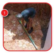
Level the ground which will form the base for the tank. Excavate the virgin solid ground. Do not use excavated material to achieve a level platform. The tolerance allowed is 40mm
