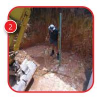
The base should be a 4 meters x 4 meters square hole x 1.9 meters depth for 3.7m 0 tanks.
