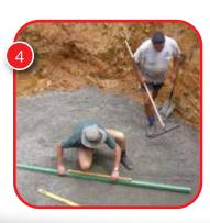
Add 7mm GAP Granular Fines as bedding material - this should be 75mm thick. Do not compact, this should be screeded to within 5mm tolerance over the entire base.
