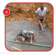
Add 7mm GAP Granular Fines as bedding material - this should be 75mm thick. Do not compact, this should be screeded to within 5mm tolerance over the entire base.
