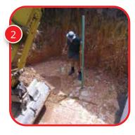
The base should be a 2.8 meters x 2.8 meters square hole x 1.9m depth for 2.5m ø tanks.
