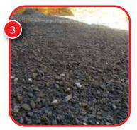
Add hard fill and compact with a compactor. Compact to a depth of 100mm thick. The tolerance to be within 15mm.
