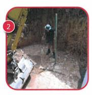
The base should be a 4 meters x 4 meters square hole x 2.275m depth for 3.7m ø tanks.
