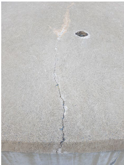
Roof Crack
