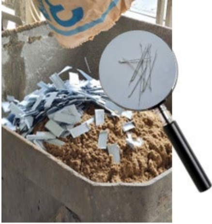
Our Steel Fibre technology being introduced to the mix
