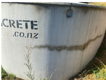
Natural curing / seeping
